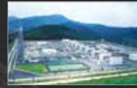
Electro Electric Systems Division
